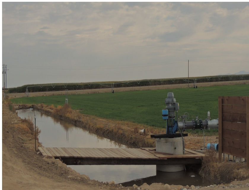
Pump Station for Pivot Sprinkler
