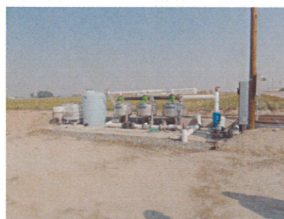
319 Tour Best Management Practices -- Sand Media Filters for an Irrigation Drip System
